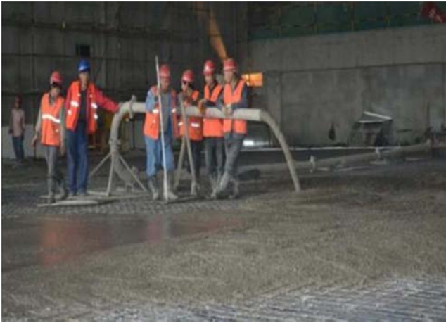
Figure 3. Construction of the ice hockey hall.
